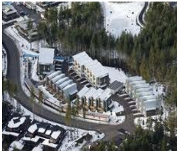
District Energy Utility
